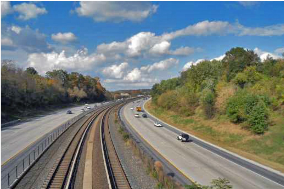
Northwest Expressway, I-795, Facing North, Parcel 336 on Right
